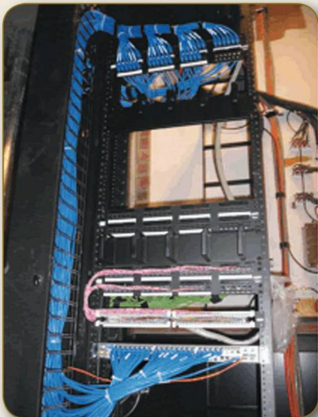
A distribution rack on each floor of the hotel sends wired and wireless Internet signals to each guest room on the floor.
